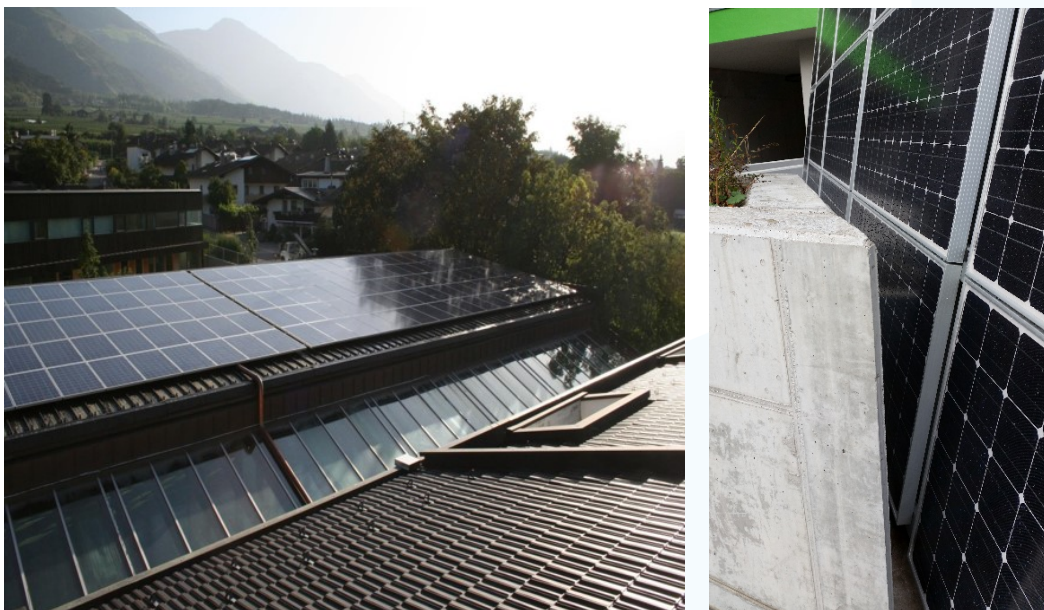
Figure 10: Example of shading due to nearby objects. Left : (tree). This type of shading is seasonal depending on foliage. Right : shading due to bad planning
